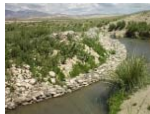
Figure 3. One of the canals in satisfactory condition
