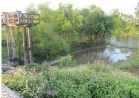
Picture 1. The gate of a ditch gets water from Nhue river for irrigation in agriculture.
