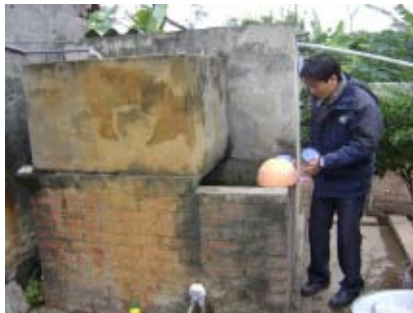
Photo 1. Sand filter with tube-well in Chuyen Ngoai, Duy Tien district, Hanam.
