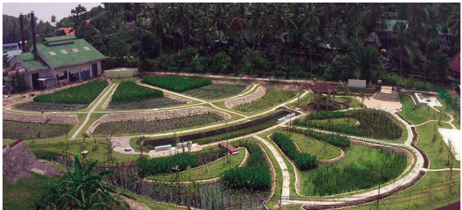
Photo 1: Constructed wetland system treating domestic wastewater of hotels and households on Phi Phi Island, Thailand. The park-like system is frequently visited, thus supporting the acknowledgement and dissemination of the technology. (Photo: T. Koottatep)
