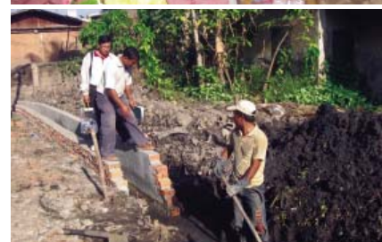
Photos 1–3: Different project phases, from top to bottom: Poor sanitation services were a priority issue for the community; Village Environmental Unit defining management regulations; construction of the stormwater drainage network. (Photos: A. Morel)
