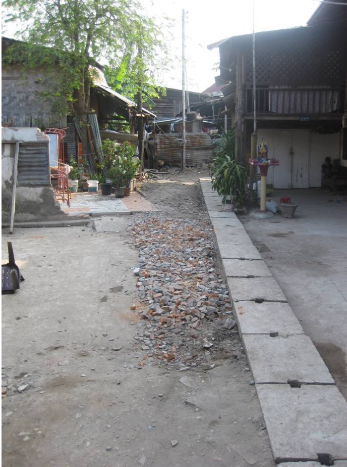
Figure 2.9: New stormwater drainage in Hatsady. (Photo: Sandec)
