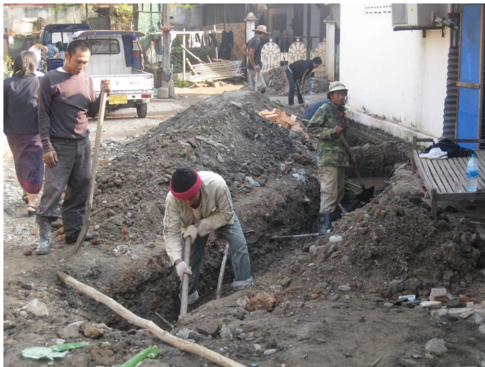
Figure 2.8: Construction of new infrastructure without heavy machinery. (Photo: Sandec)
