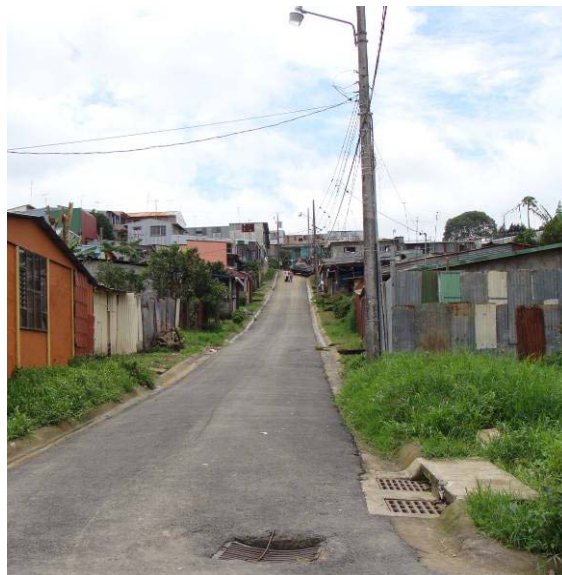
Figure 5.7: Asphalted main road with stormwater drains. (Photo: Sandec)
