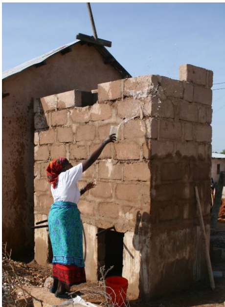
Figure 4.11: Construction of pilot urine-diverting toilet for awareness raising purposes. (Photo: Sandec)
