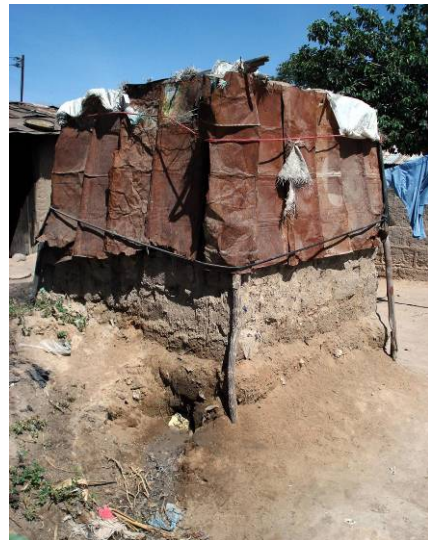
Figure 4.8: Existing unimproved pit latrines in Chang'ombe. (Photo: Sandec)
