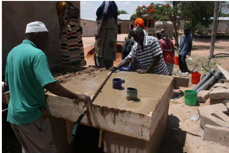
Figure 6.2: Building of demonstration Ecosan toilets in Chang'ombe, Dodoma. (Photo: Sandec, December 2008)
