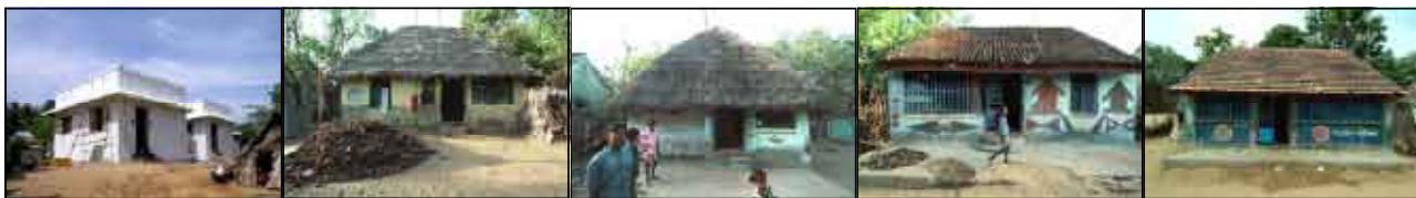
Type 1 – RCC flat roof Type 2 – coconut thatched roof Type 3 – straw thatched roof Type 4 – hand made tiles roof Type 5 – Mangalore tiles roof
