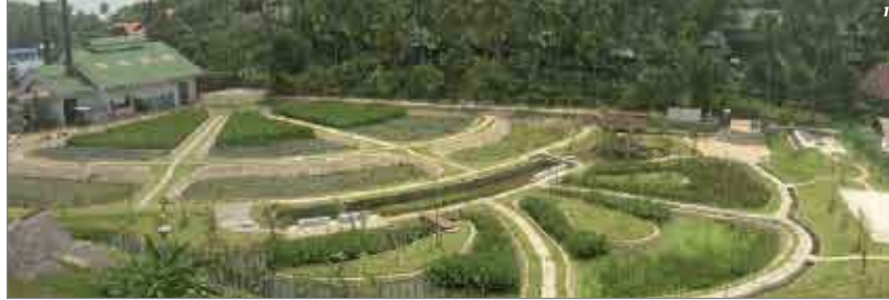
Figures 1-3: Constructed wetland system treating domestic wastewater of hotels and households on Phi Phi Island, Thailand. The park-like system is frequently visited, thus supporting the acknowledgement and dissemination of the technology. (Photos by T. Koottatep)
