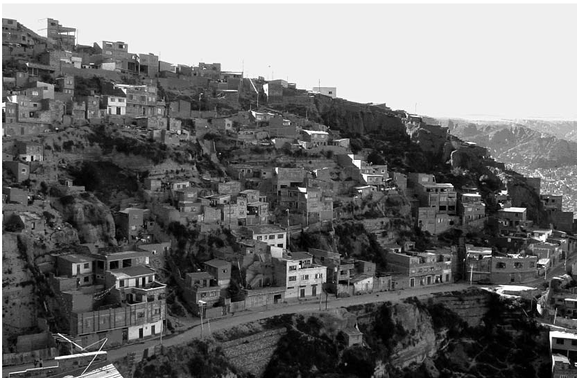
Fig. 2 Dangerous slopes in La Paz. (Photo by Fabien Nathan)
