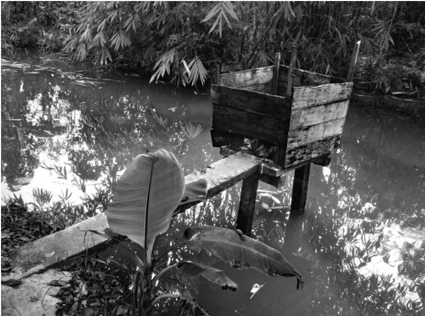
Fig. 3 A typical hanging latrine over a fish pond in a peri-urban community in Cantho city, Vietnam. (Photo by Thammarat Koottatep)
