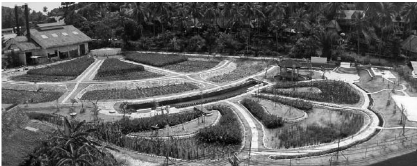
Fig. 2 Constructed wetland system treating domestic wastewater of hotels and households on Phi Phi Island, Krabi Province, Thailand. (Photo by Thammarat Koottatep, 2007)
