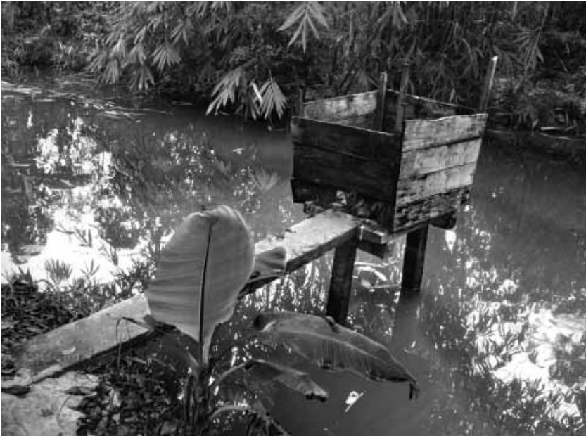
Fig. 3 A typical hanging latrine over a fish pond in a peri- urban community in Cantho city, Vietnam. (Photo by Thammarat Kooattap)
