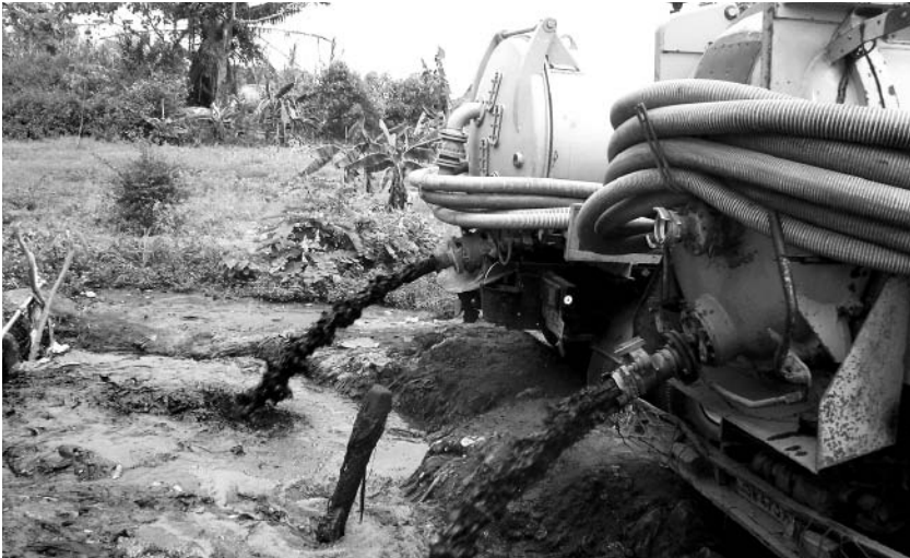
Fig. 1 Anarchic discharge of faecal sludge from on-site sani- tation systems in Cameroon. (Photo by Ives M. Kengne)
