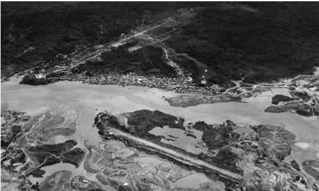
Fig. 2 View of Huepetuhe ( Wepetwe means "place of jaguar" in Harakmbut). (Photo by FENAMAD)
