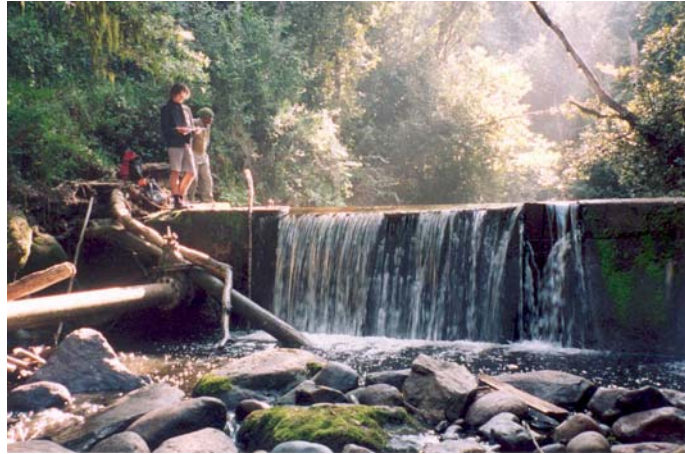
Fig. 2.12: The weir at the intake of Gitwe Water Project on Naro Moru North. The gravity pipe, with a sluice gate to control the flow, is visible on the left side (Picture by J Aeschbacher).
